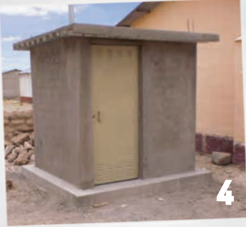
The shed was built out of cinder blocks, following the plans and norms provided by Technical Assistance.
